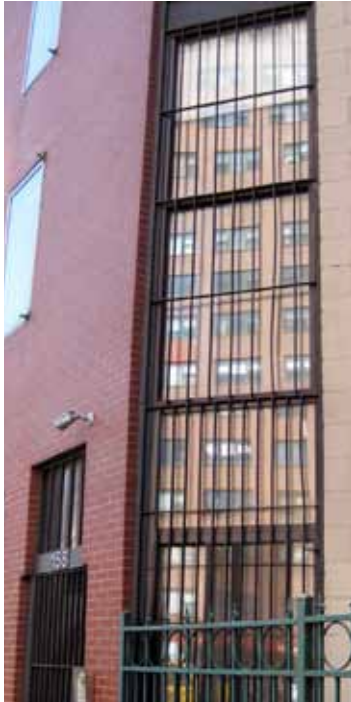
This security grille creates a pattern that will deter birds from flying to reflections. Photo: Christine Sheppard, ABC
