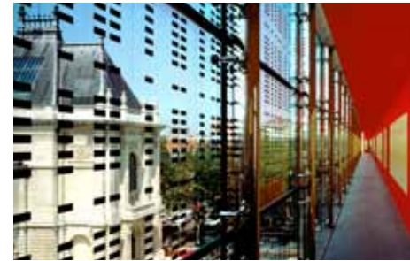
External frit, as seen here on the Lila Museum of Fine Arts, by Ibos and Vitart, is more effective at breaking up reflections than patterns on the inside of the glass. Photo: G. Fessy
