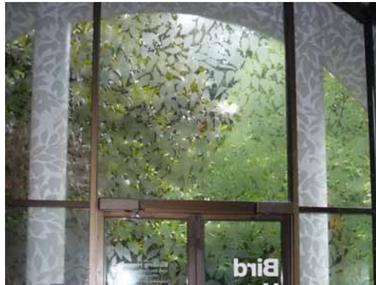
Patterns achieved with film or by etching glass can be beautiful as well as very effective in preventing bird collisions. Photo: Bob Sallinger
