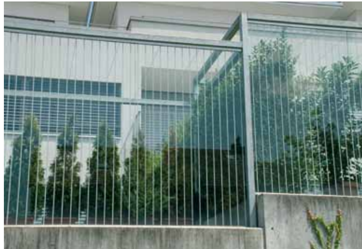
The white stripes on this glass wall are an easy way to make a very dangerous area safe for birds. Photo: Hans Schmid
